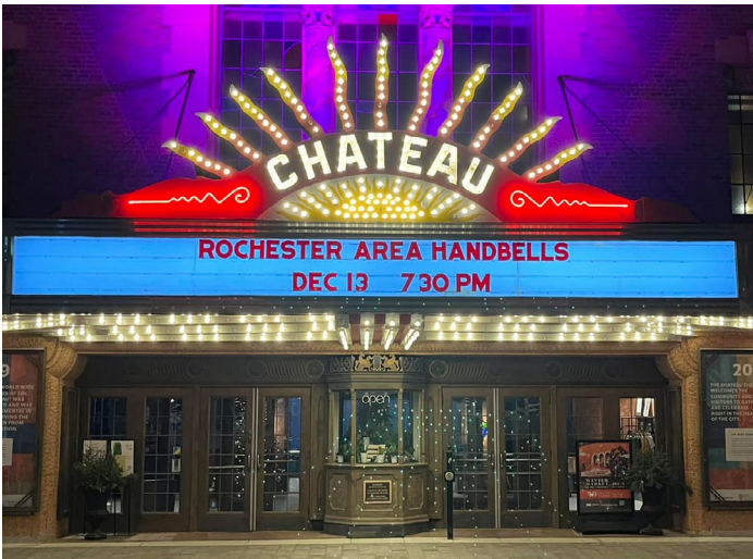
Lighting up the night — our first marquee!
